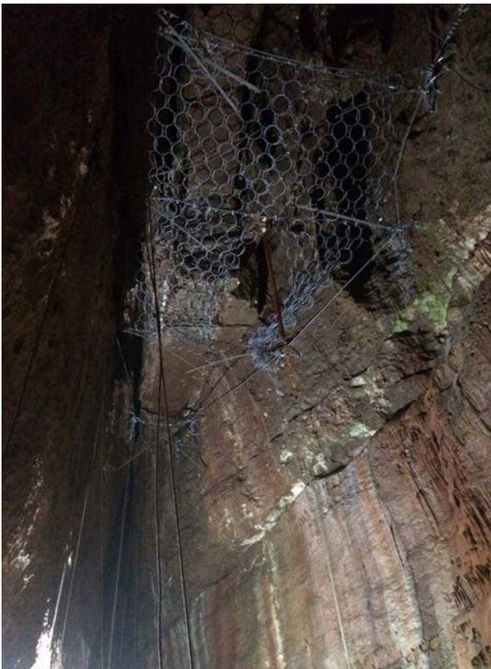
Above: Catch net during construction, note the presence of two smaller panels about to be joined together. This was done to allow the panels to be carried in to the caves by hand.
