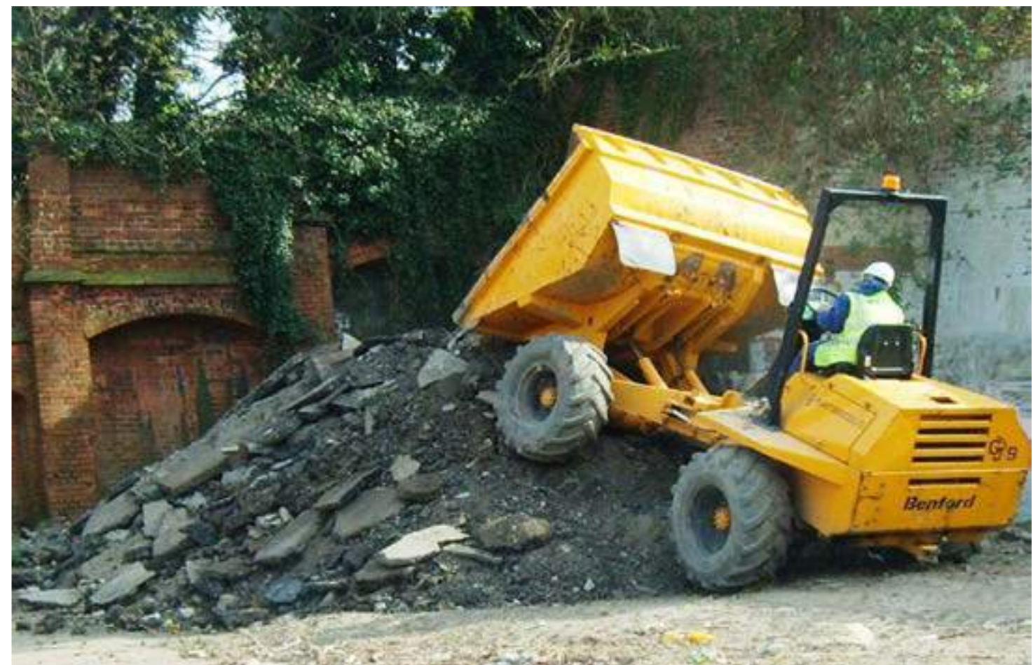
Stockpiling of waste tarmac on a construction site (courtesy of James Stokes – DTS Raeburn)
