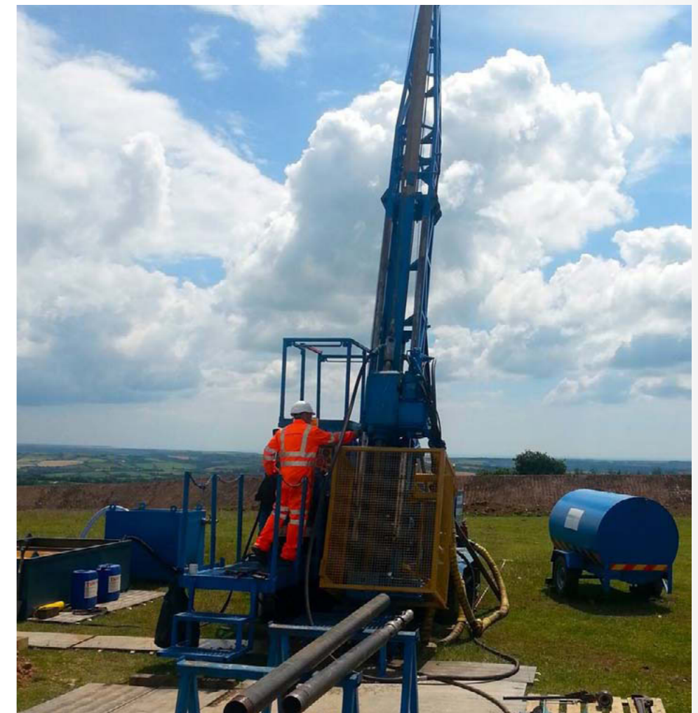
Geotechnical: The Meridian team used an Atlas Copco CS14 rig, which was customized for the project.
