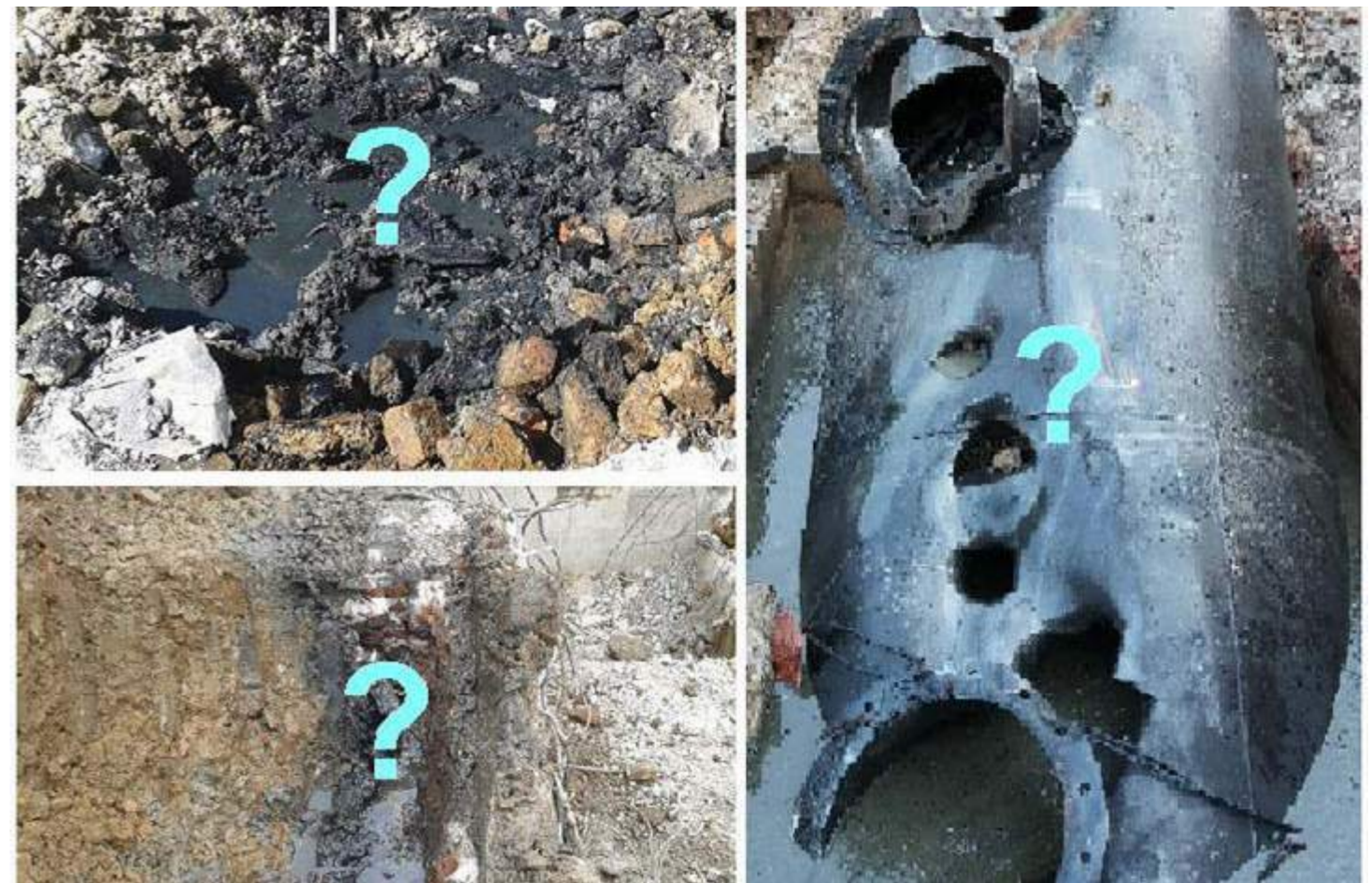
Unknown contaminants and tanks found on a site. Image courtesy of James Brown, DTS Raeburn.
