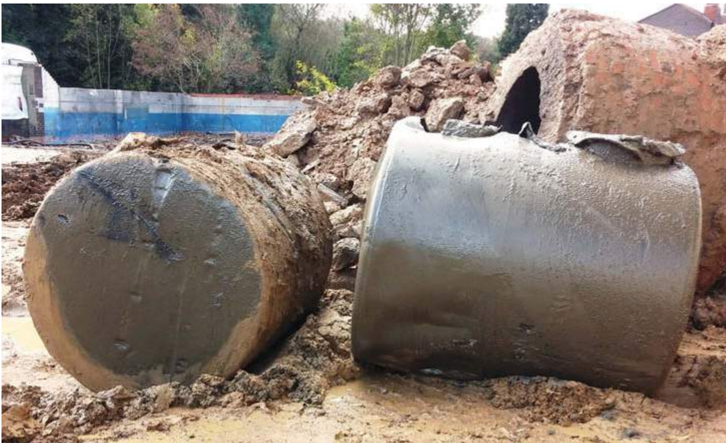
Underground storage tanks found at a site with limited historical information. Image courtesy of James Brown, DTS Raeburn.
