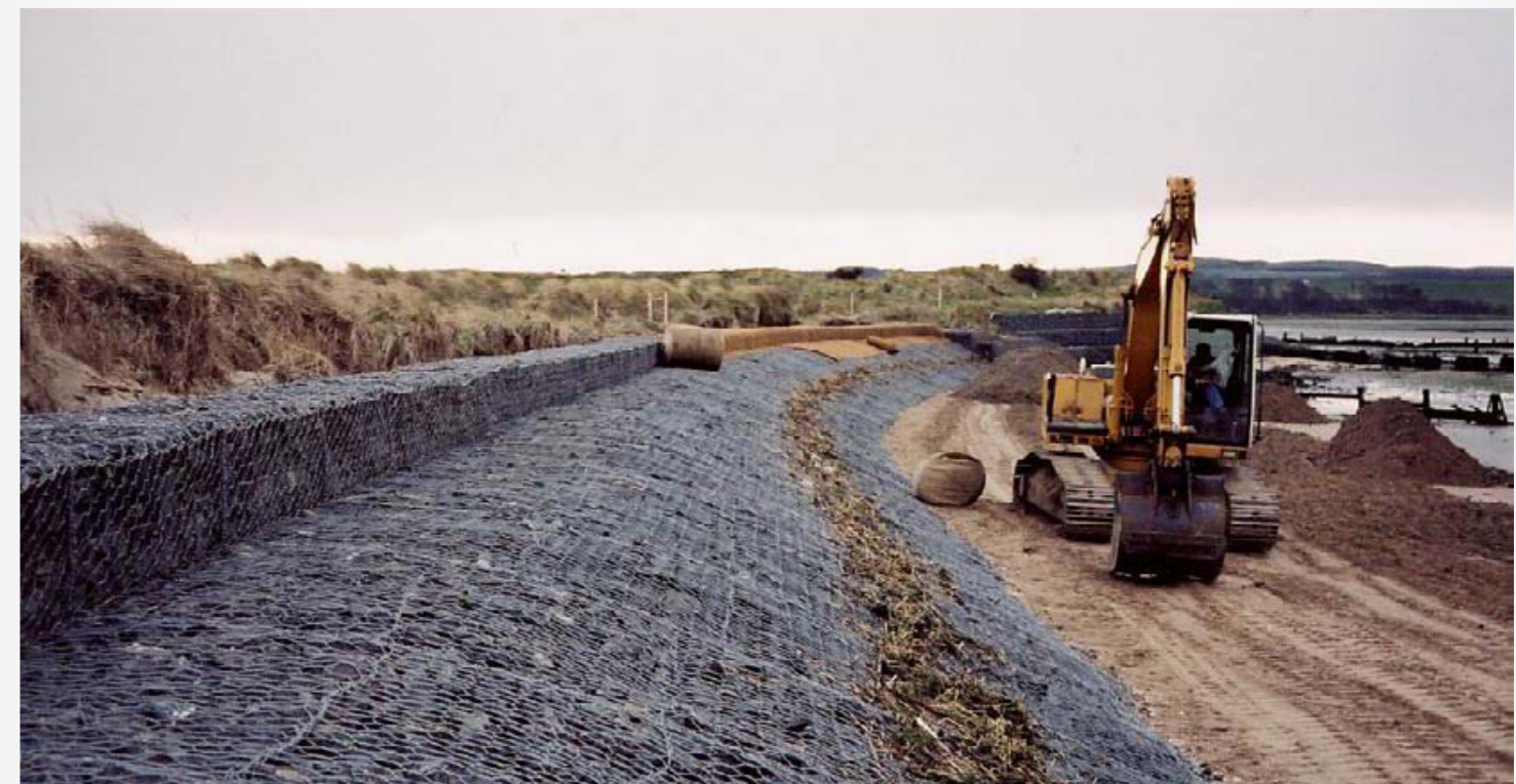
Maccaferri Gabions and Reno Mattresses were used to reinforce vulnerable beach and dune areas adjacent the world famous St Andrews links golf course in Scotland.
