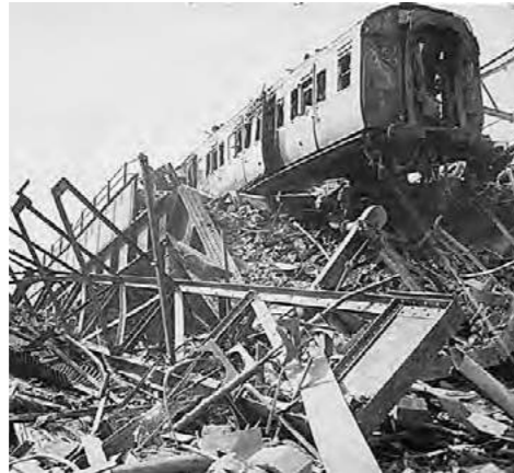
Major targets: Rail infrastructure.
