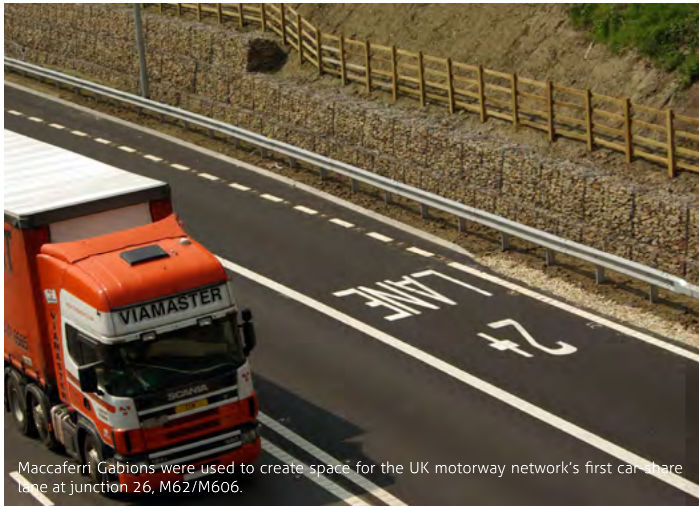
A huge slender, free-standing Maccaferri Gabion wall – thought to be the biggest in the UK - has been built to screen outdoor filming areas at the BBC Roath Lock studio in Cardiff.
