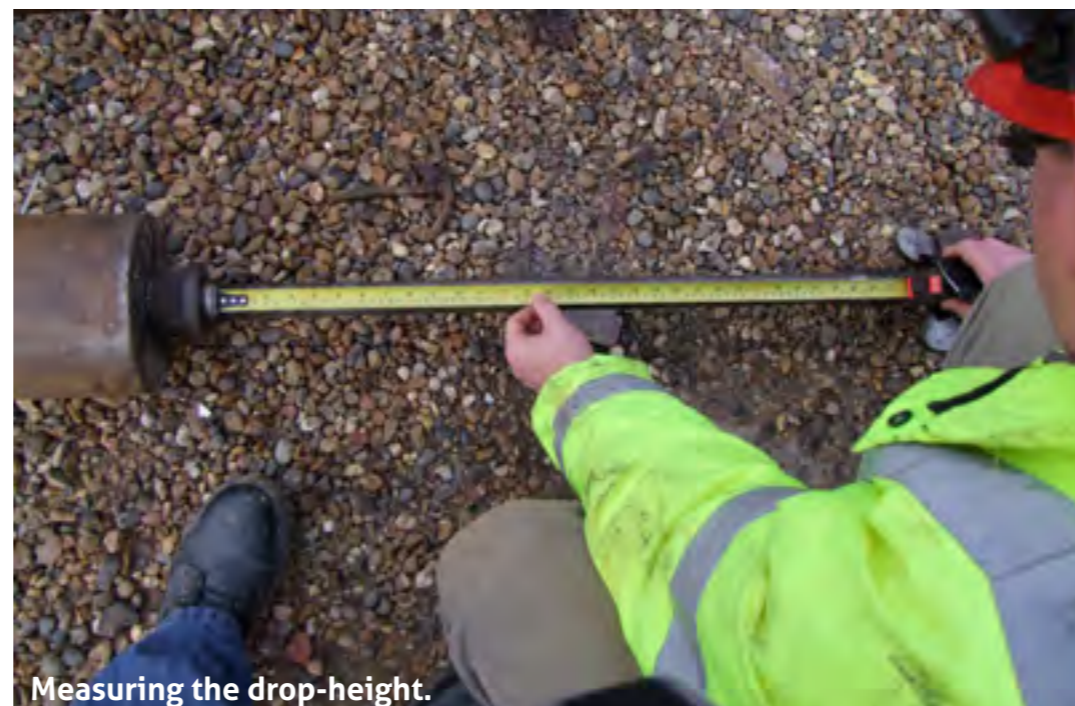
An SPT Calibration on a Cable Percussion rig.
