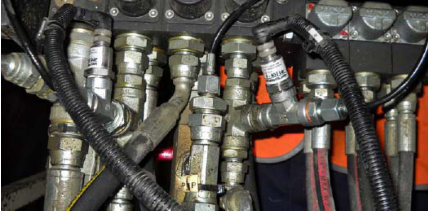
Pressure sensors on the TBM.
