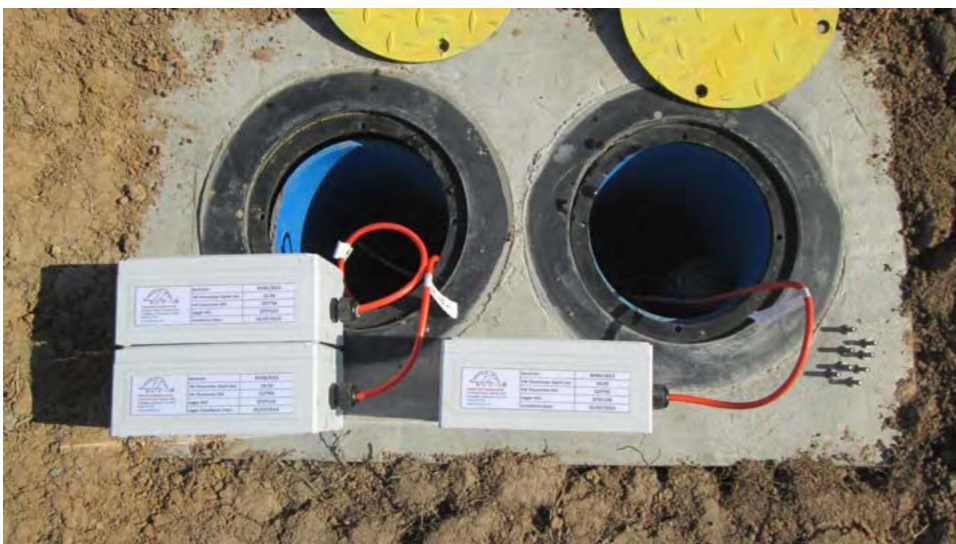
Installations at the Barton on Sea site
