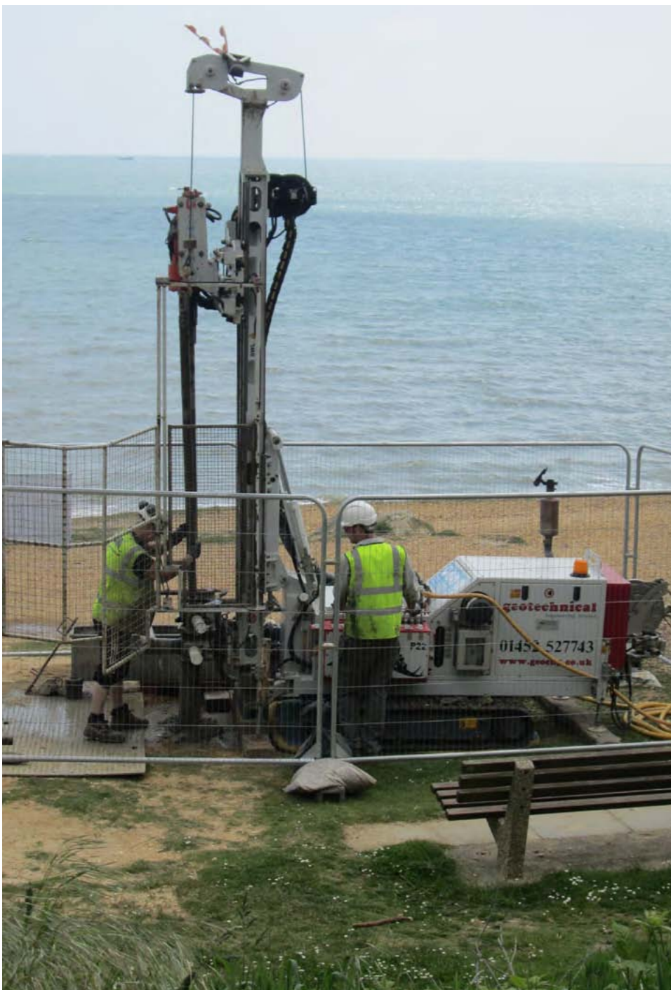
Geotechnical Engineering drilling technicians
